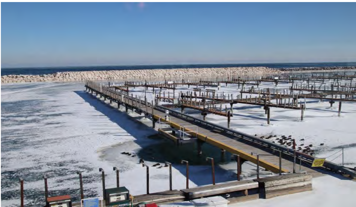
Finished layer of smooth stone applied over the new wider base.
