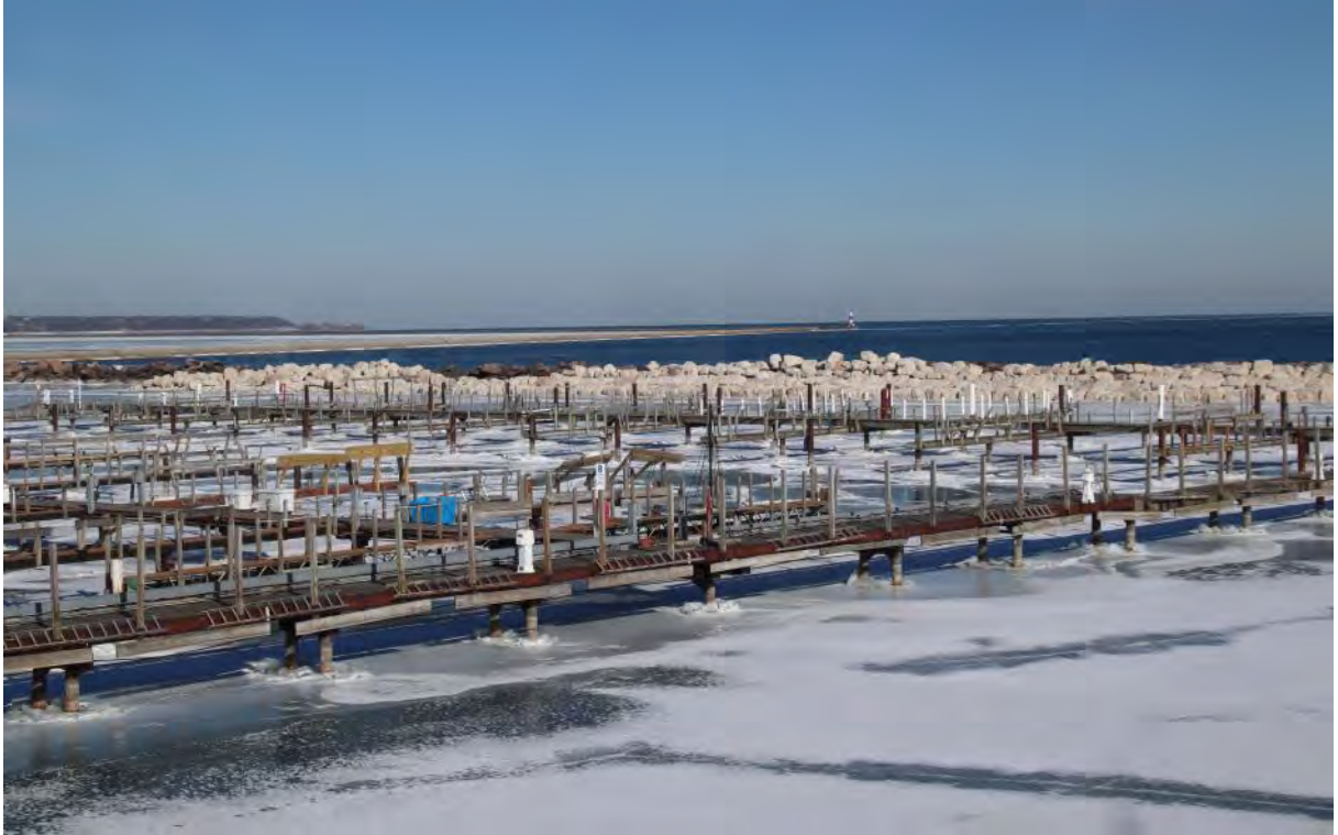
Breakwater being raised with fresh rocks and fill
